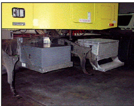
Figure 1. Box Holding Deep-Cycle Batteries
